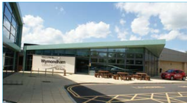
Wyomdham Leisure Centre GMV5 Heat Recovery UK
