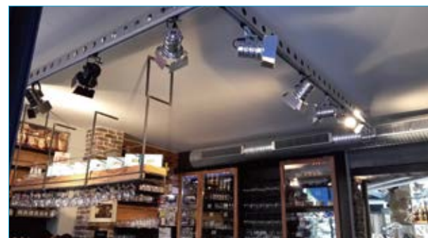
Trattoria Restaurant U-Match; Duct France
