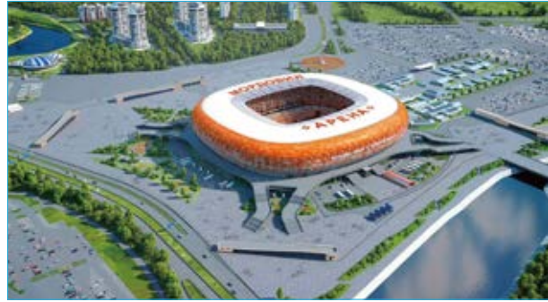
Mordovia Arena Water-cooled Screw Chiller; Fan Coils Russia
