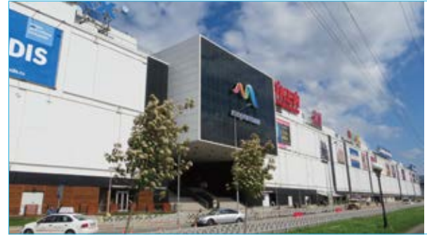
Sochi More-Mall Centrifugal Chiller Russia
